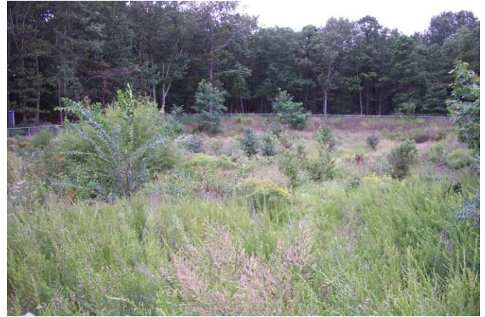
Bay Avenue Basin now drains within 48 hours of a rain event due to the benefits of Soil Health restoration. Water is able to infiltrate through the soil because soil is no longer compacted and vegetation has become established. Ocean County Soil Conservation District has identified 3500 basins within the county.
